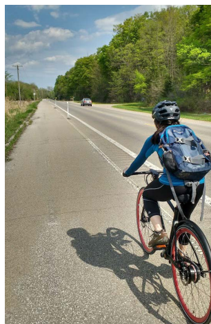
This paved shoulder with a buffer in Cambridge, Ontario, provides a link between two off-road recreational trails.
