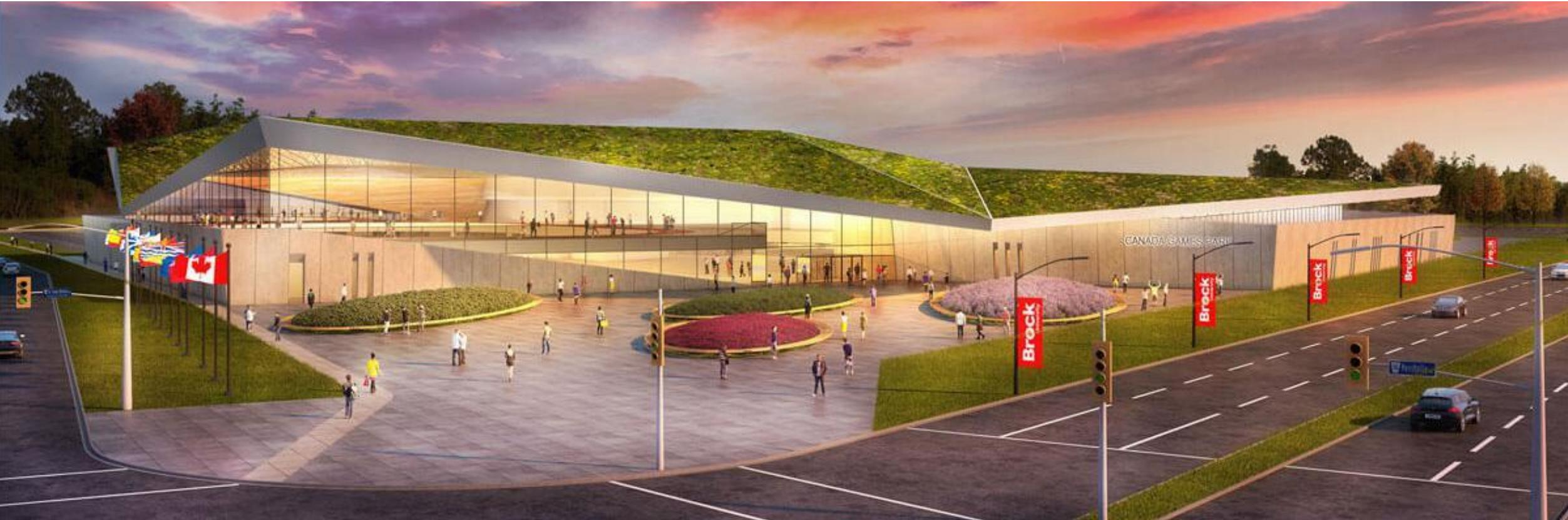
The “green roof” will help control stormwater and the urban heat island effect while reducing energy costs, and that’s made possible by the way the building was designed – 35% more efficient and generating 45% less GHG emissions than standard buildings.
